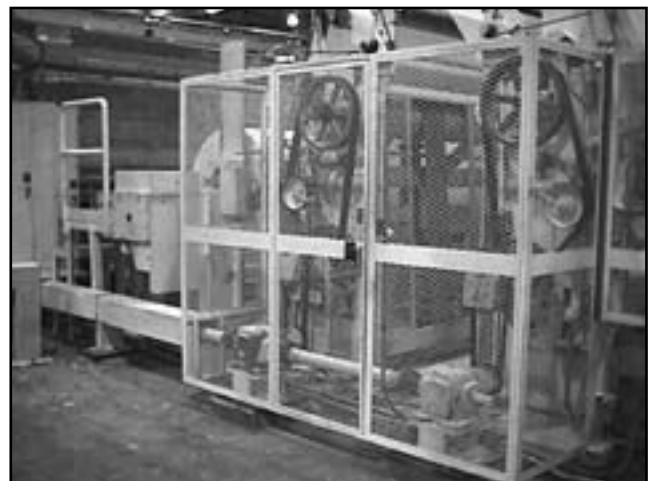
Fixed guard enclosing several belt drives.
